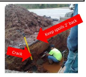
EVEN "SHALLOW" TRENCHES ARE DANGEROUS. EVEN THOUGH THIS IS A "SHALLOW" TRENCH, THIS EMPLOYEE COULD BE SERIOUSLY INJURED BY THE WEIGHT OF THE FALLING SOIL. IN THIS PHOTO THE SPOIL PILE IS TOO CLOSE TO THE TRENCH EDGE AND THE SIDE WALL IS CRACKING.
